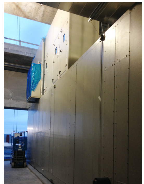
One of the two large Ventrol heat recovery units being installed during construction
