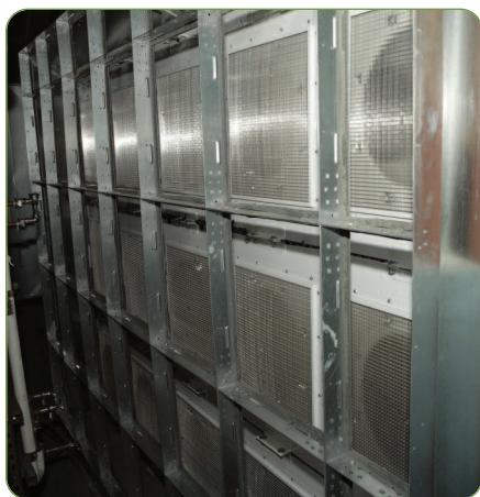
Inlet side of one 5x3 FANWALL array with inlet screen shown. Screen helps to reduce preswirl of air entering the fan and reduces sound levels.
