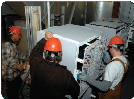
FANWALL cells are easily stacked together to form a 5x3 array.
