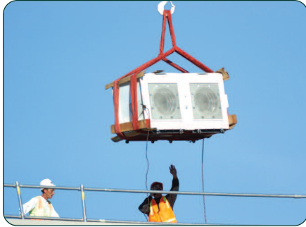
FANWALL cells are lowered by crane into the penthouse equipment room.
