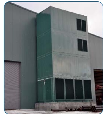
Two air handlers, each delivering 62,000 cfm, were designed to be stacked as four sections, simplifying transportation and site erection.
