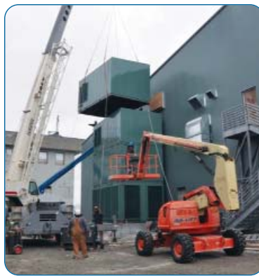
Two air handlers, each delivering 62,000 cfm, were designed to be stacked as four sections, simplifying transportation and site erection.
