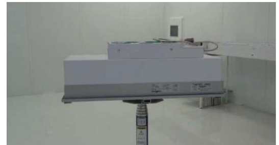
Figure 2. FFU shown on top of lifting hoist.
